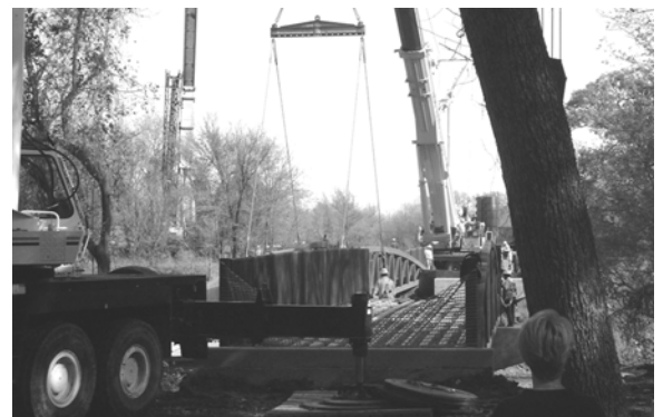
Last November workers installed the central section of what must be Arlington's most impressive pedestrian bridge.
