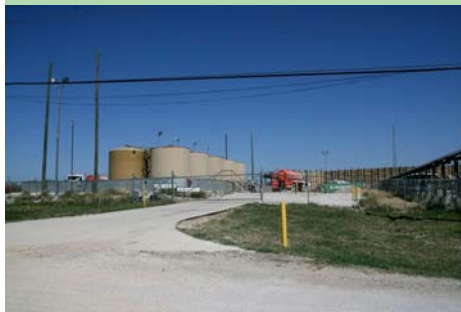
Tanks holding the waste water and gas byproducts from the compression process.
