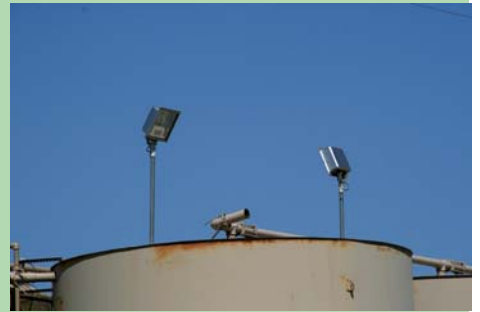
Closeup of a safety valve on top of the tanks that lets gasses escape as the liquid in the tanks heats up on a hot day.
