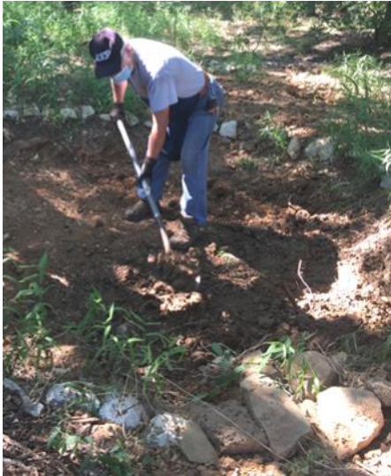
Joe Martinez led the excavation for two rain gardens.
