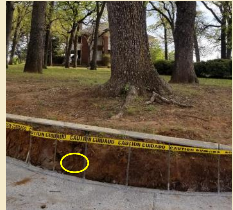
Fielder House post oak closest to new sidewalk. Circle shows location of two large severed roots.
