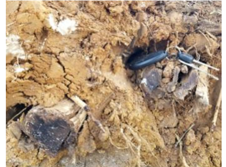
Two large post oak roots severed for a sidewalk on north edge of Fielder House Museum property.
