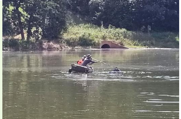
Workmen replacing fountain pump July 7, 2021. Photos by Carol Marcotte.
