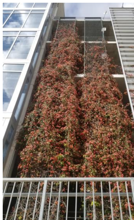
Cross vine, UTA parking garage
