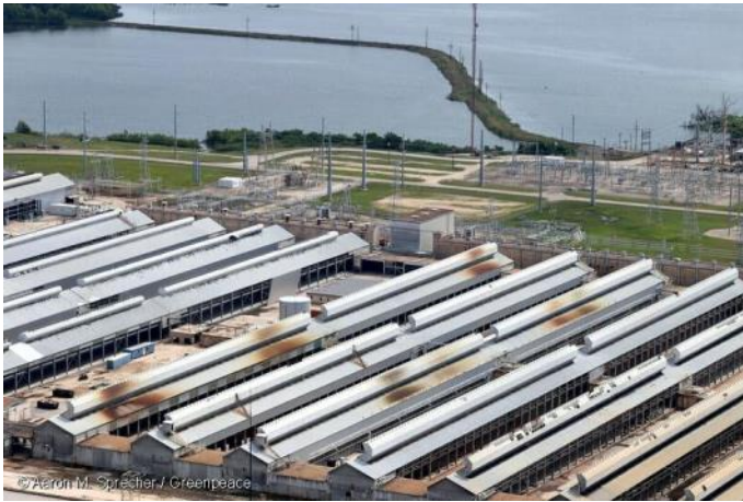
Riot Platforms facility at Rockdale, Texas
