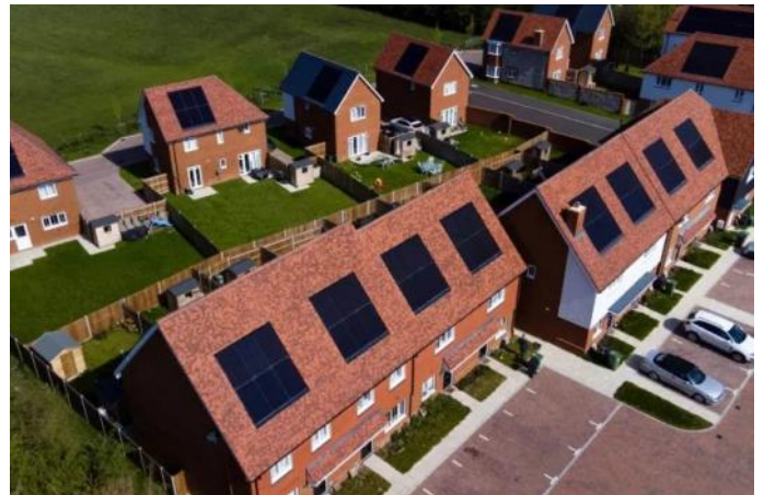
Above, Solar panels on new homes in the UK.
