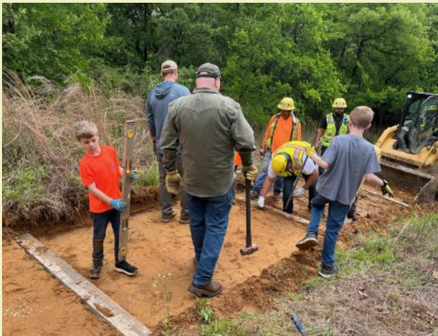
Above, Yellow Trail restoration with timbers by SouthPoint Constructors volunteers in April. Jim Fuquay photos. Below, Jim Frisinger (yellow shirt) and Rudy Arnold use decomposed granite to resurface the Blue Trail. Jim Domke photos.
